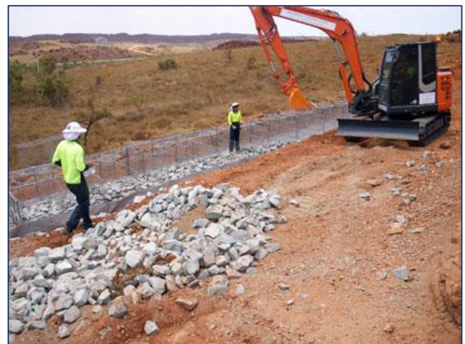
Figure 3-Example of Gabion Installation
